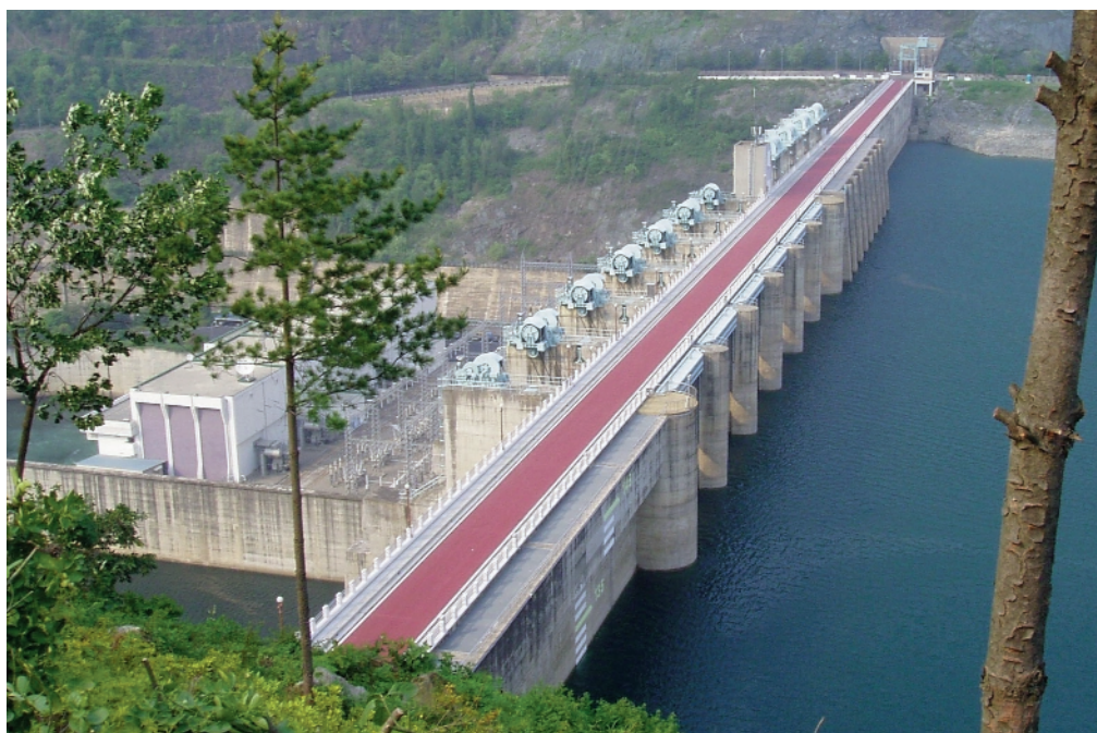
Chungju Multipurpose Dam, South Hangang River, Korea.
